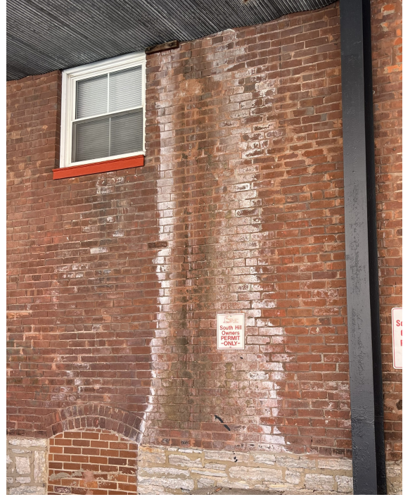
Exhibit 4: Moisture of Brick Wall
