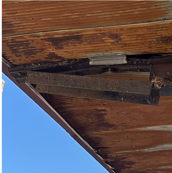
Exhibit 5: Altered Steel Beams
