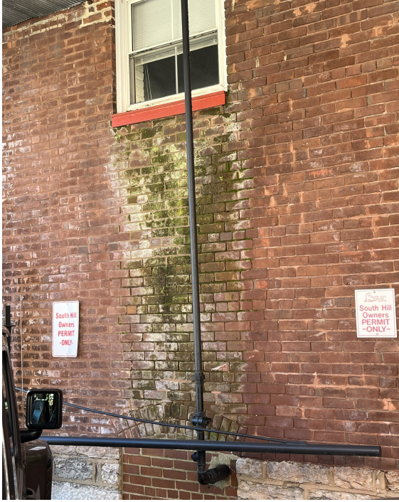
Exhibit 4: Moisture of Brick Wall
