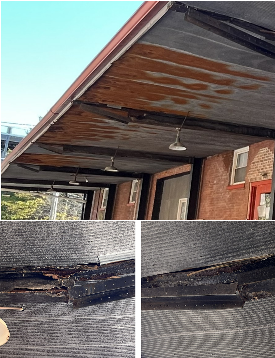
Exhibit 7: Rusty Awning Decking and Beams
