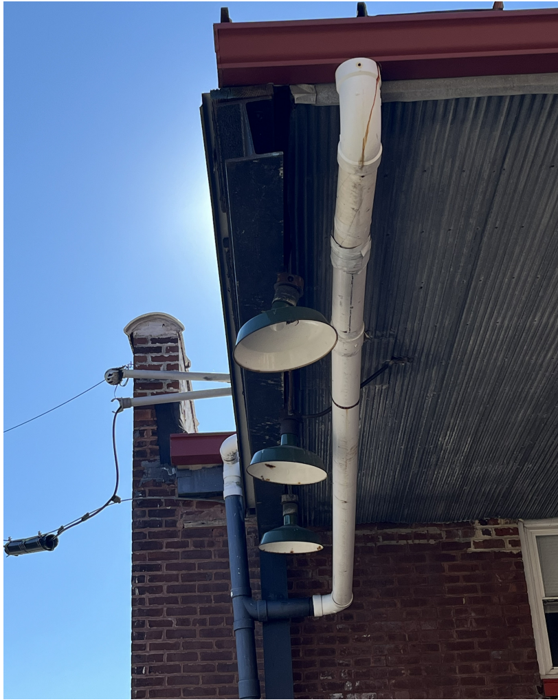
Exhibit 6: Out-of-Level Beam
